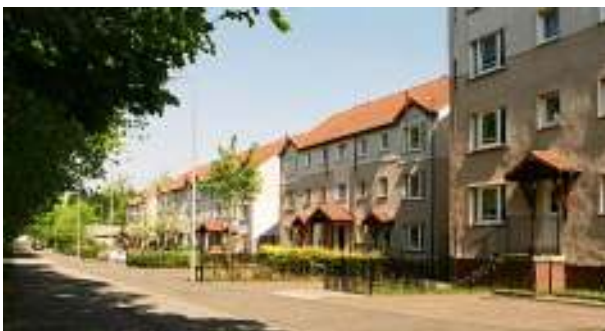
Our improved flats looking down Davaar Drive
